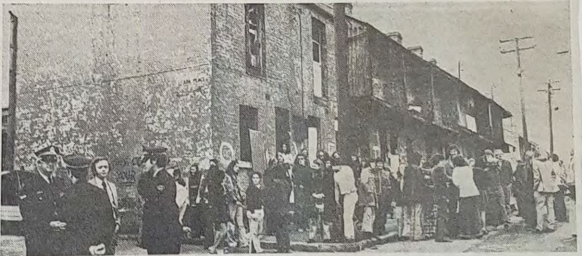
A crowd of people gathers outside the houses in Fig Street. The Department of Main Roads is clearing the way for the Western Distributor.
